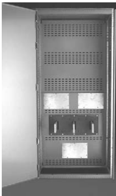
Optional rear main bus barriers, providing a completely isolated cable compartment.
