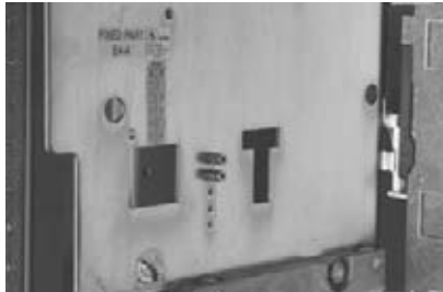
Emax breaker rejection feature.
