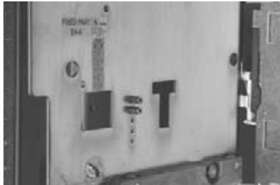
Emax breaker rejection feature.
